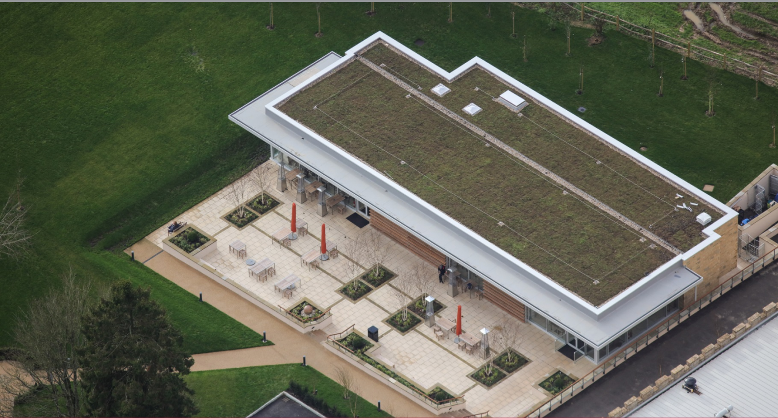
VerdiRoof installation on the café in Sussex
