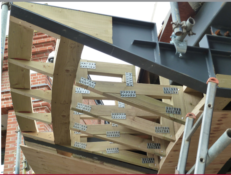
A slim steel structure with a ring beam portal frame helps to create a 6m overhanging canopy clad in SIG's copper sheeting
