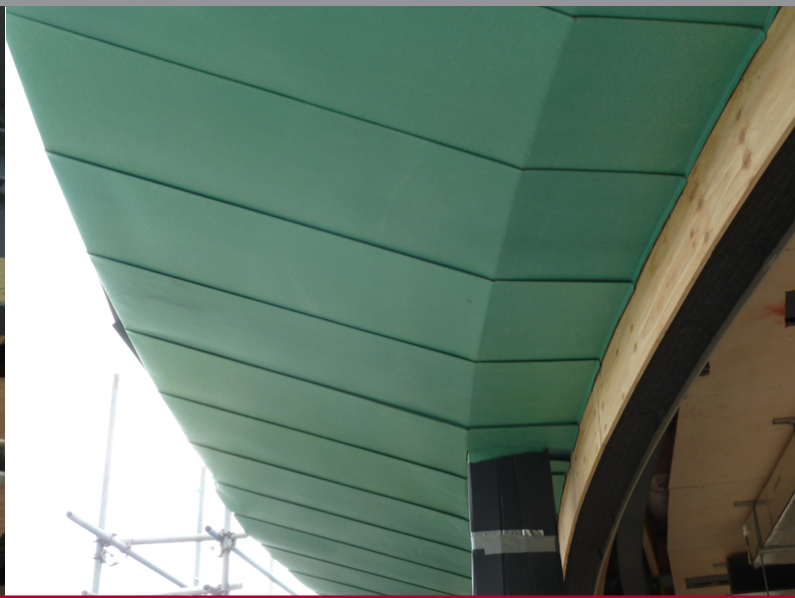
A slim steel structure with a ring beam portal frame helps to create a 6m overhanging canopy clad in SIG's copper sheeting
