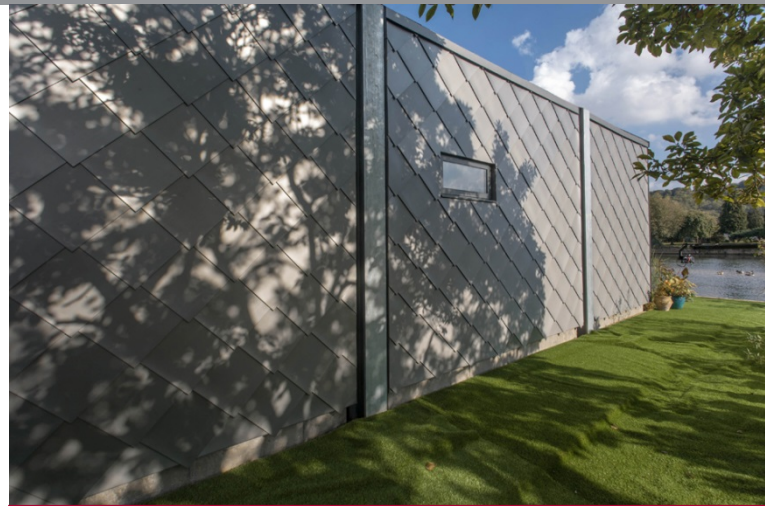
Rooflights follow the line of the dolphins creating a challenging ventilation detail. Photo © Tim Crocker
