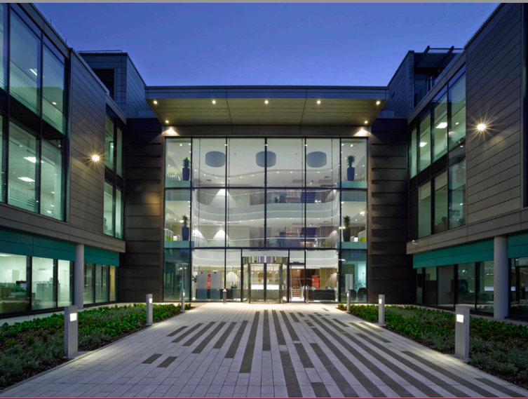
The versatility of zinc is clear at Imperial Tobacco's Bristol HQ, where it moves from roof to façade to become a smart coat that will withstand all weathers. Designed by AWW Inspired Environments
