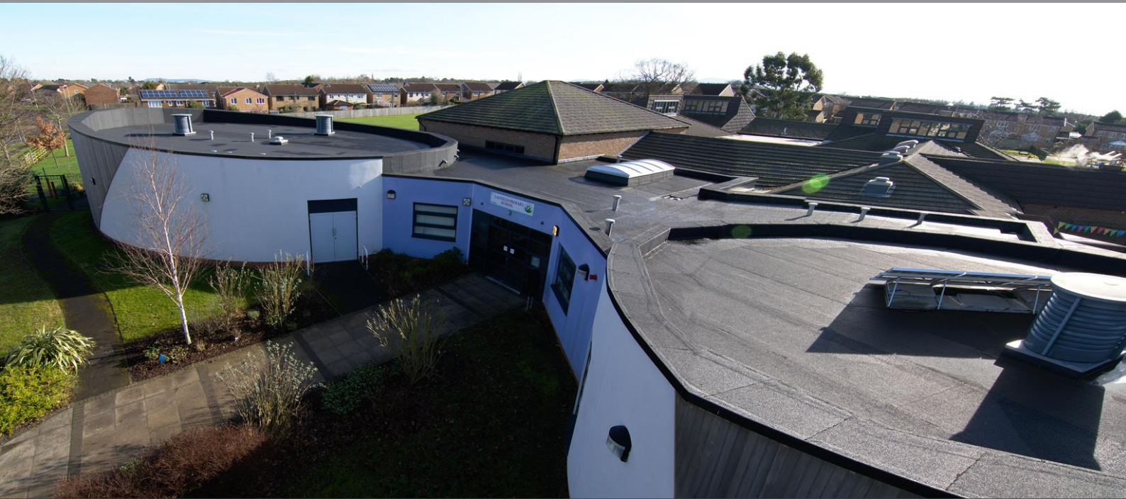
The new overlaid roof at Layfield Primary
