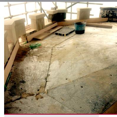
Hydrostop AH+ was used as an alternative to lead traditionally used on buildings of this age - due to its ability to be used on a shallower pitch.
