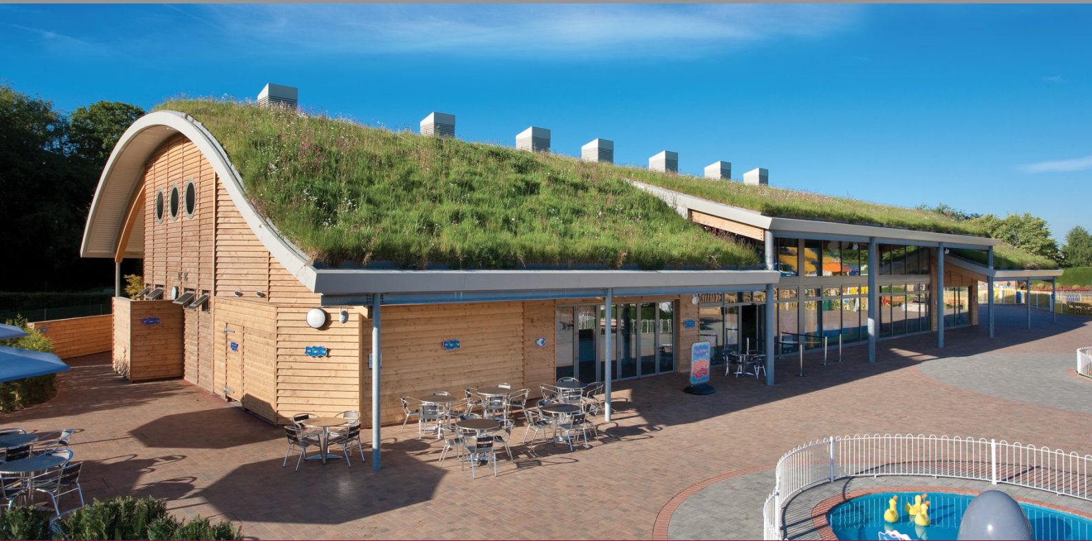
Peppa Pig World's main building from the front, neatly tucked under its wildflower turf roof.
