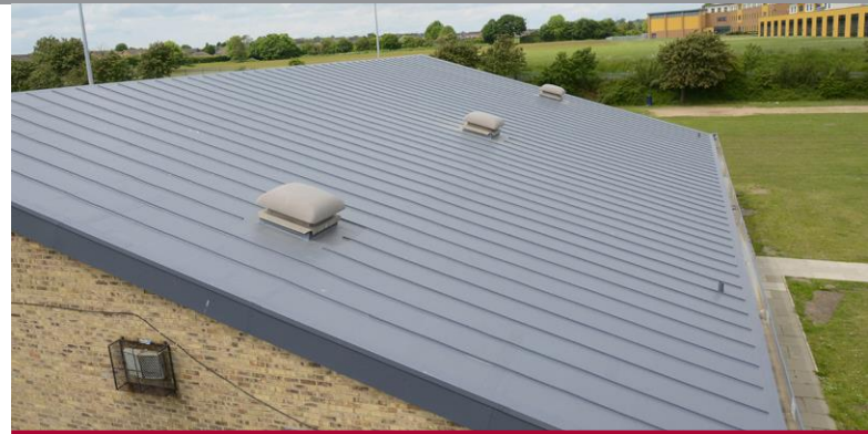
The swimming pool waterproofed with Armourplan PSG standing
