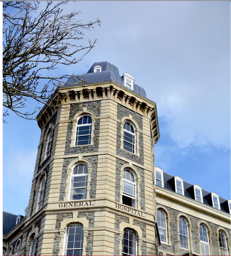
City & Country were granted planning permission on the condition they could recreate a key feature of the Bristol General, the distinctive Ogee Dome
