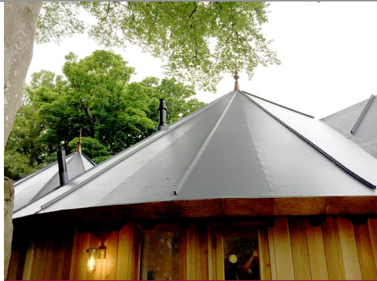
A single ply membrane with excellent sustainable credentials plus the added benefits of the seam profiles justified switching to a more contemporary material, Armourplan P single ply.
