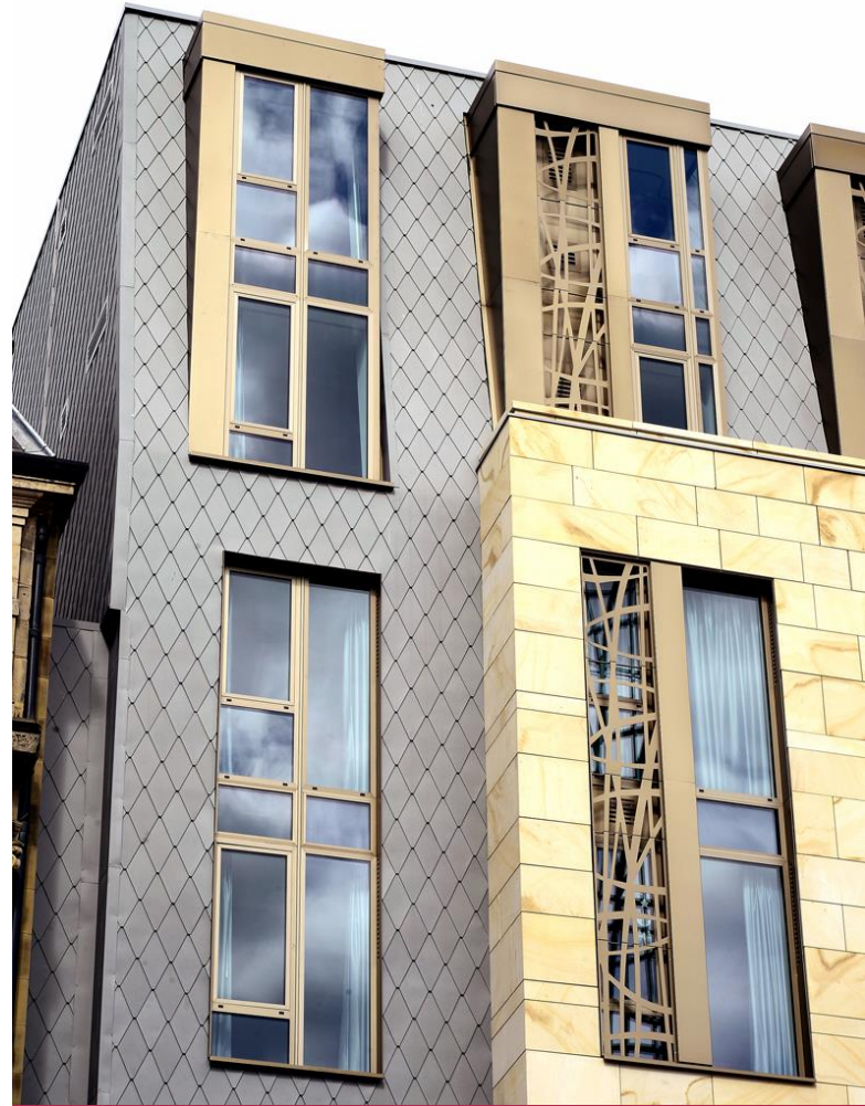
The resulting density of shingles looks extremely attractive next to the anodised aluminium perforated screens and provides an appropriate foil to the neighbouring 19th Century buildings
