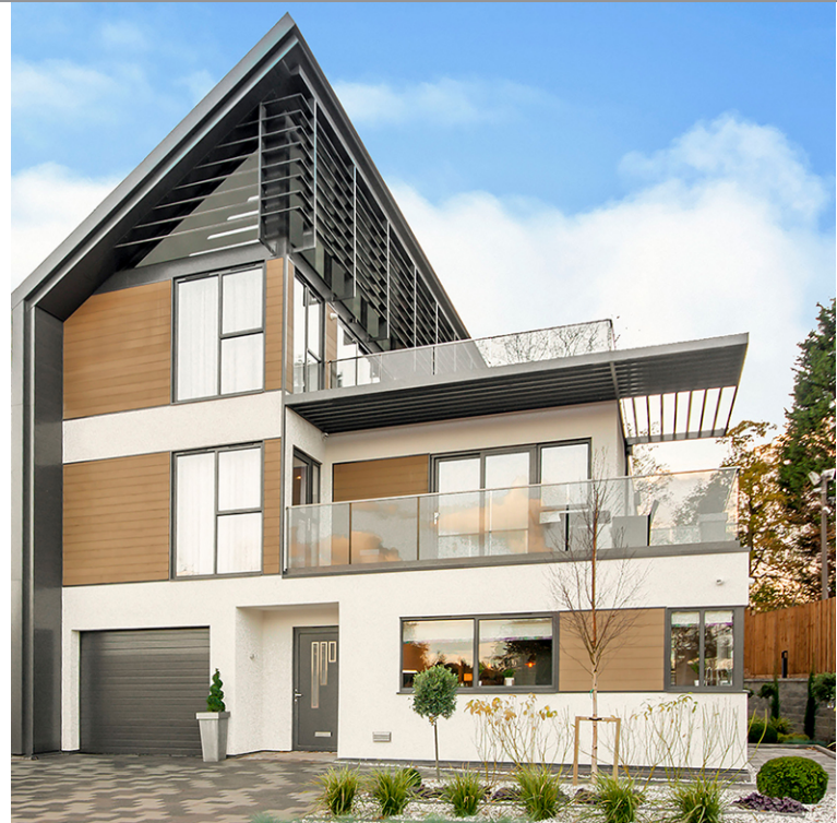
The front elevation presents a house of two halves, a large terraced area to one side and a striking pitched roof on the opposite.
