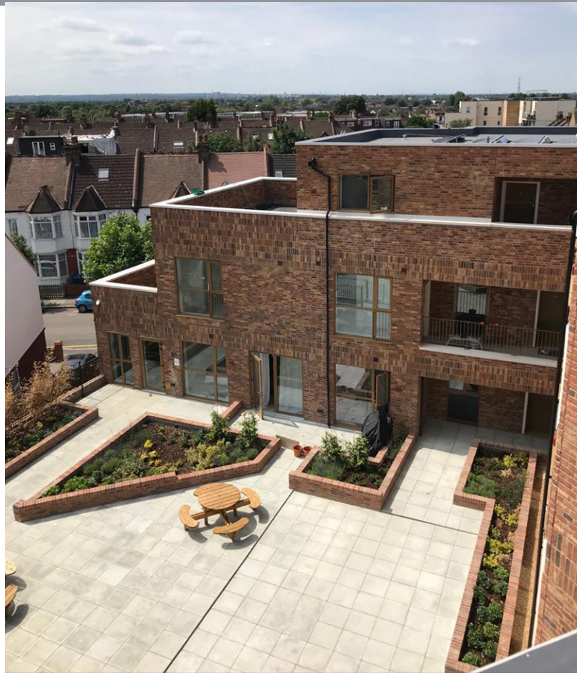
IKO Permateg was specified for the terraced courtyard and overlaid with pedestals and paving slabs.
